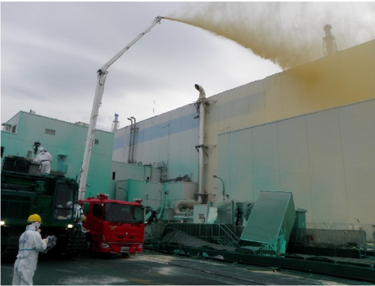
Dust Suppression Resin Application
