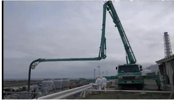
Sealing Underground Trenches
