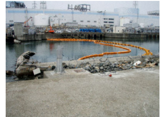
Silt Fences, To Adsorb Cs/Sr
