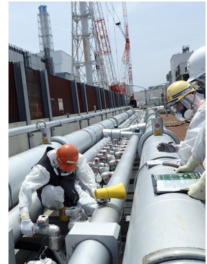
Ice wall Construction
