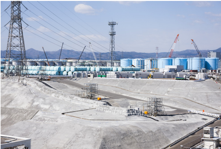
Extensive Soil Paving
