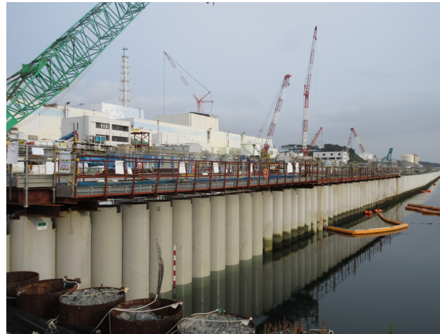
Steel Seawall Construction
