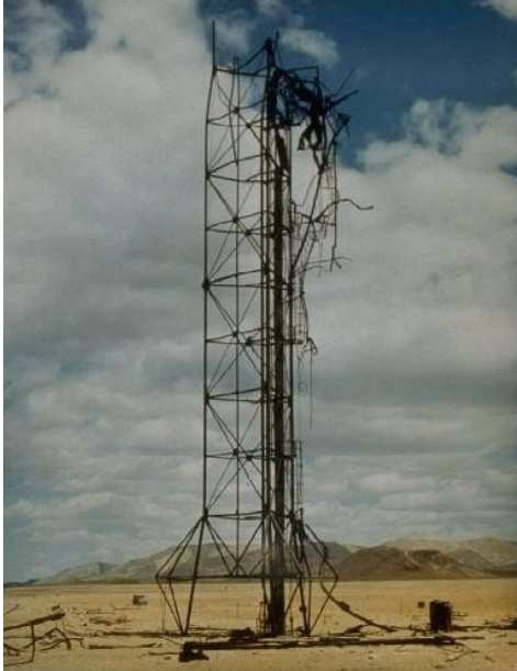
Tower from the Ruth test. The explosion failed to demolish the tower - Los Alamos referred to it in DC as the invention of the “reusable test tower”!
