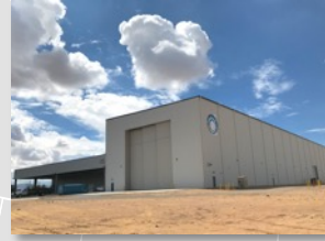
T-Facility / Engineering Test Unit Production Development Facility Albuquerque, NM
