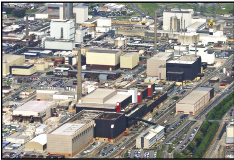
The THORP facility at Sellafield, UK, reprocessed UNF via aqueous reprocessing until 2018
