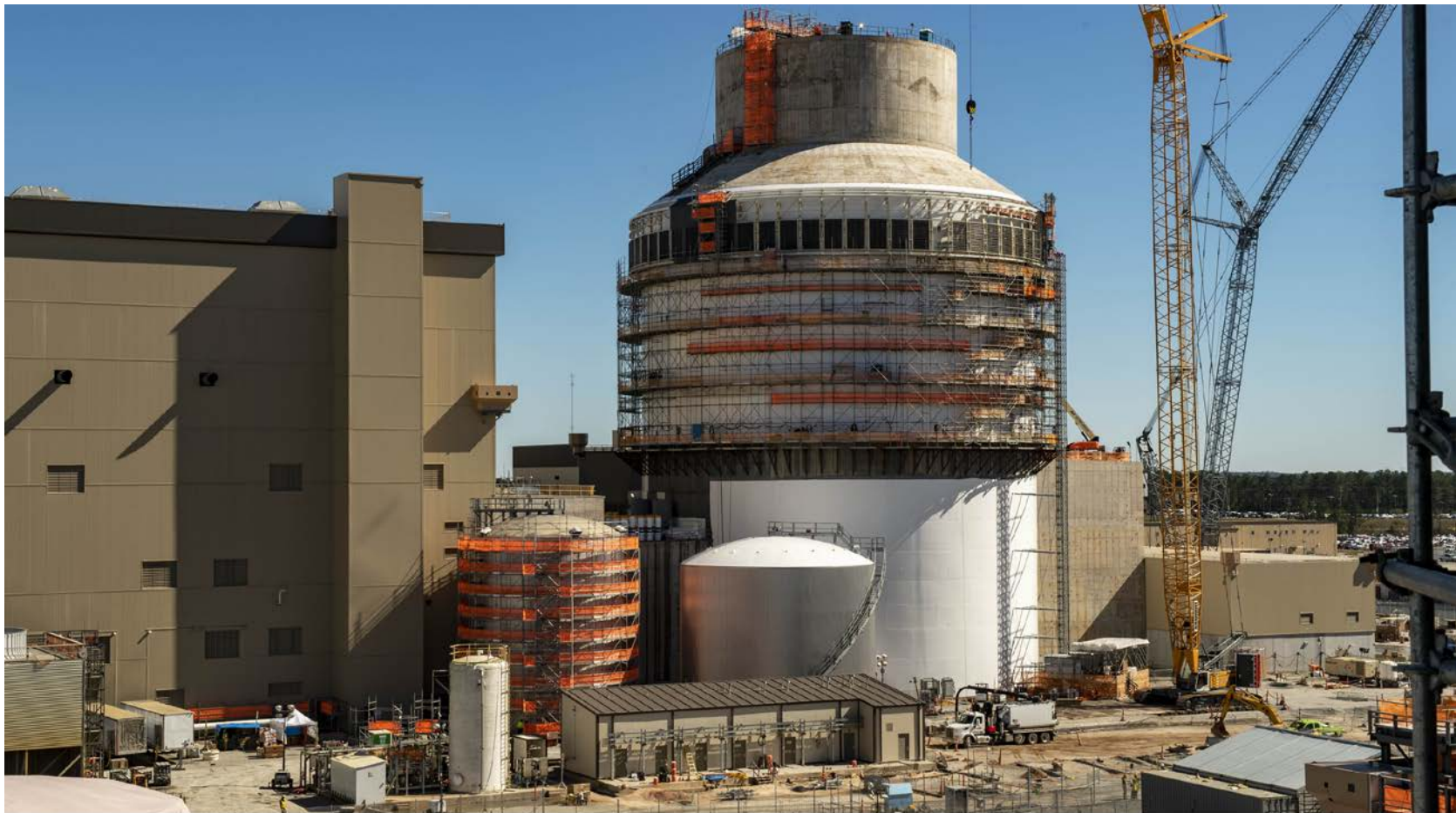
Vogtle Unit 3 Containment and Turbine Building
