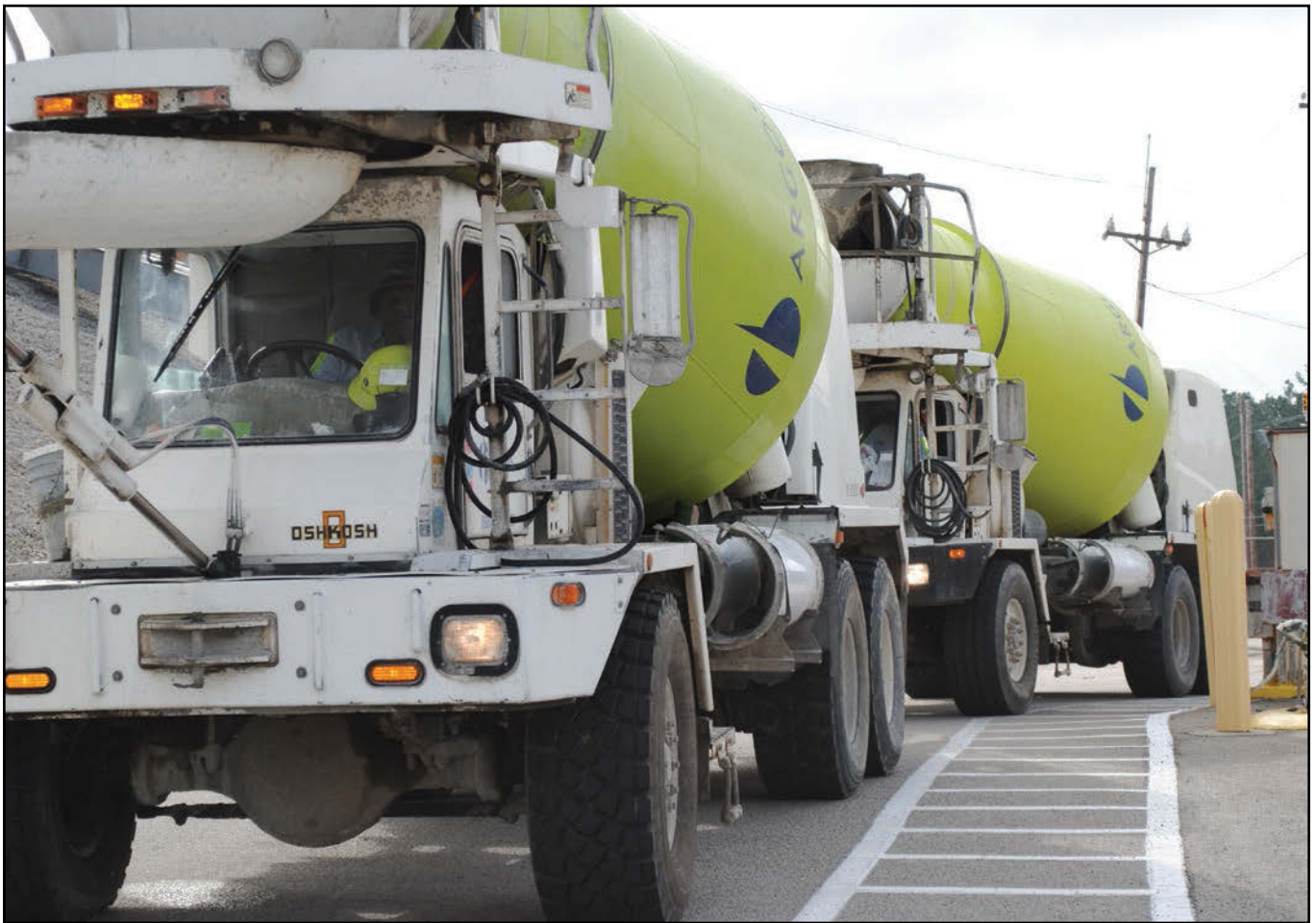
Cement trucks line up on June 2, 2015, to begin filling Tank 16 with specially formulated grout.
