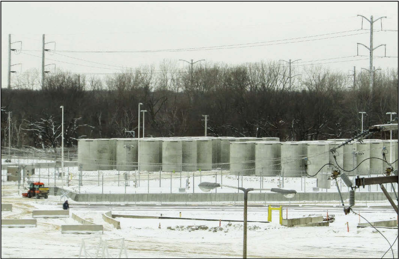
The full Zion ISFSI contains 61 Magnastor spent fuel casks and four greater-than-Class C waste casks. Other than a switchyard, the ISFSI will be the only remaining structure on the site once decommissioning is completed in 2020. ■
