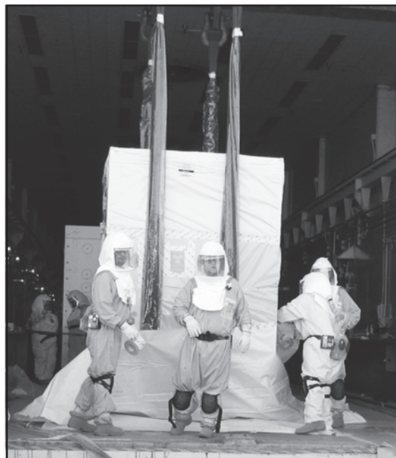
HOT CELLS WIRE SAWED FLUSH TO FLOOR
