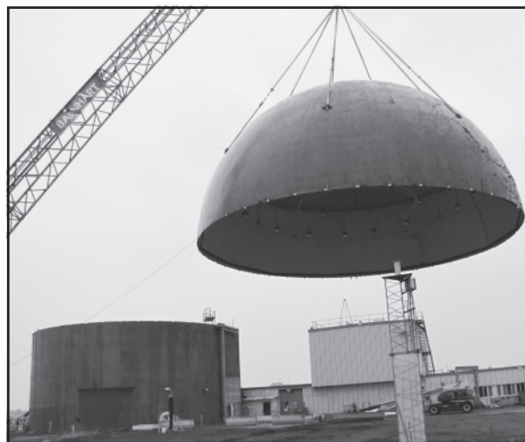
REACTOR DOME REMOTELY CUT
