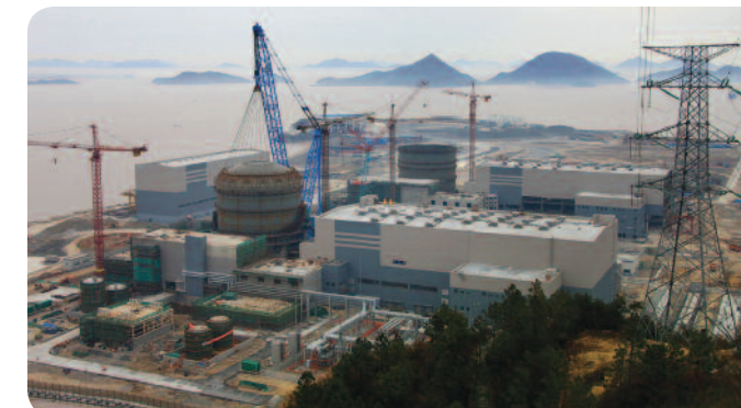
Sanmen Units 1 and 2, China
