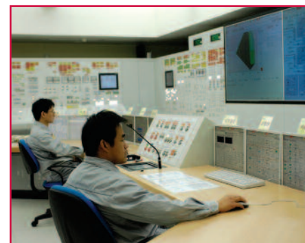
Full Scope Power Plant Simulator
