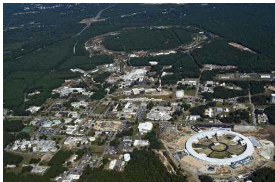
The central campus of Brookhaven National Laboratory. The National Synchrotron Light Source II, under construction at the time of this photo, is at bottom right, and the 3.8-km-circumference ring of the Relativistic Heavy Ion Collider can be seen in the distance at the top of the frame.
