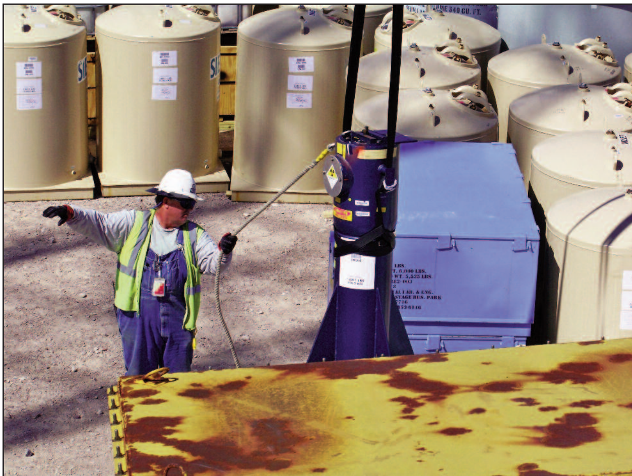
Like most LLW, RTGs disposed of at the NNSW were handled without any special equipment or clothing because of the relatively low dose rate levels.
