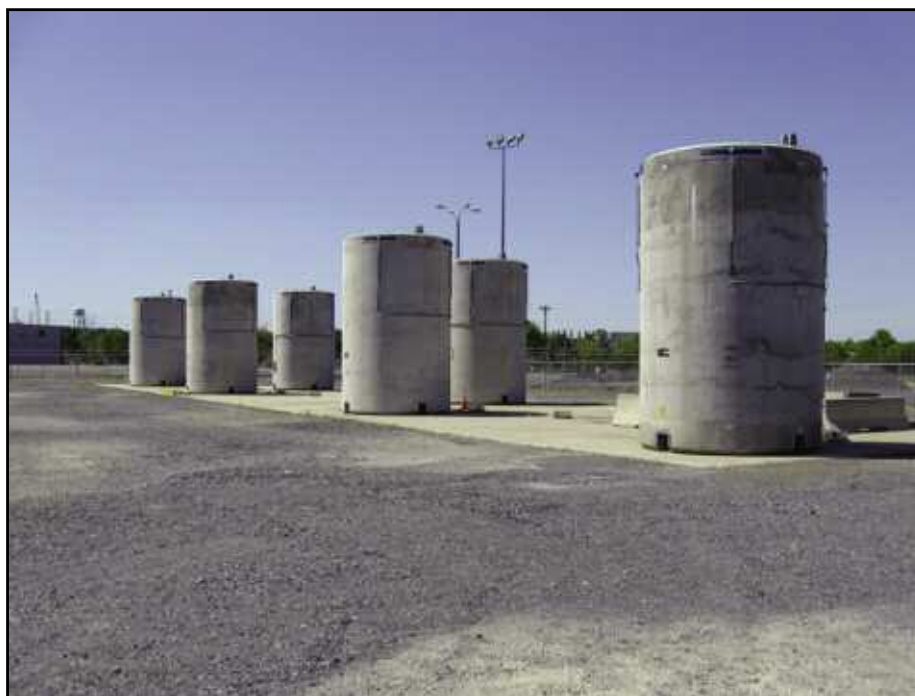
Fig. 2. Nuclear power plant onsite dry storage facility.
