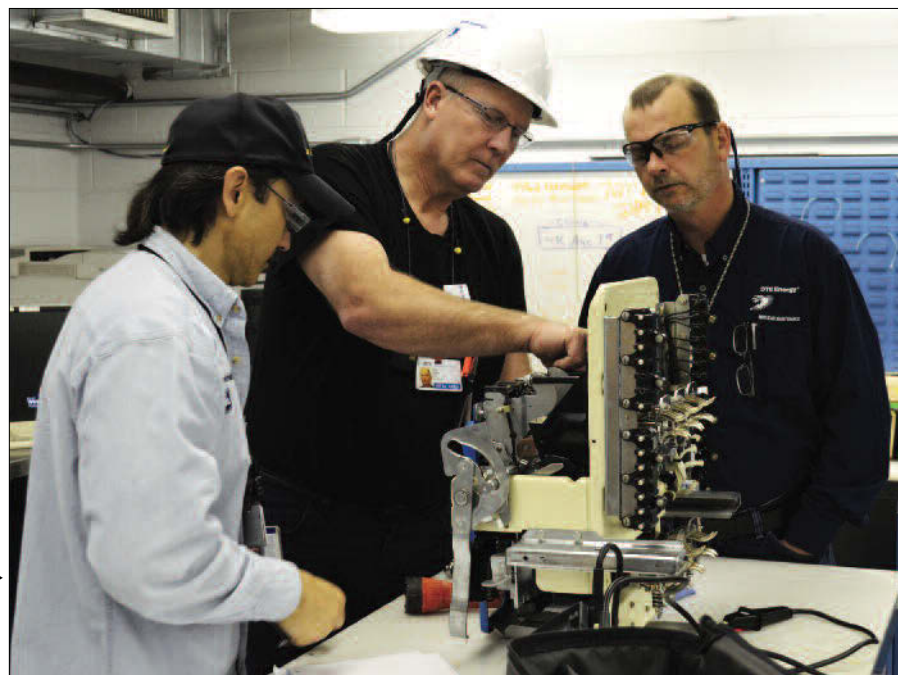
From left, Gabriel Verespec, Sam Hiner, and David Vanek perform preventive maintenance on a field circuit breaker for a motor generator.
