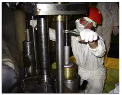
Sodium draining operations on BN-350 reactor top.
