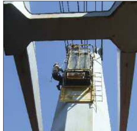
A cool shot of rather pedestrian work. See article beginning on page 46 for details.
