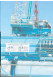
Installation, Site Services and Parts
