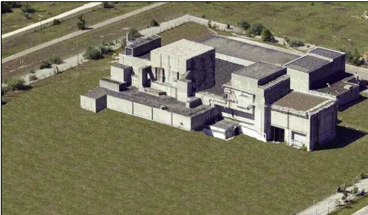
If the recommendation for in-situ P Area closure is approved through the regulatory process, the reactor building will look similar to this when work is completed.
