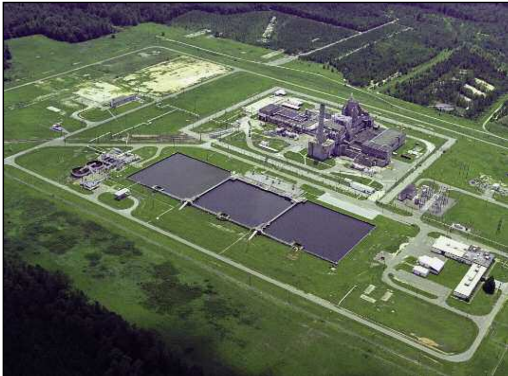
P Area as it looked in 2002, before deactivation and demolition work began in the area.
