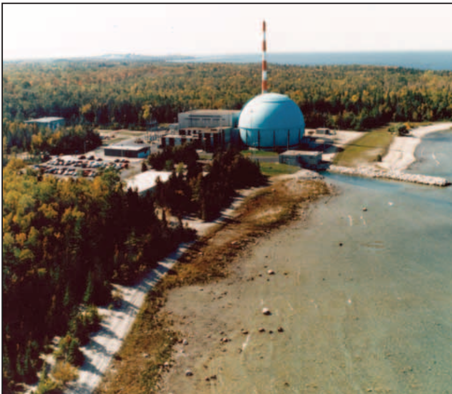
The Big Rock Point plant before start of decommissioning.
