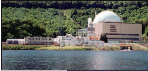
The Yankee Rowe plant before (above) and after decommissioning.
