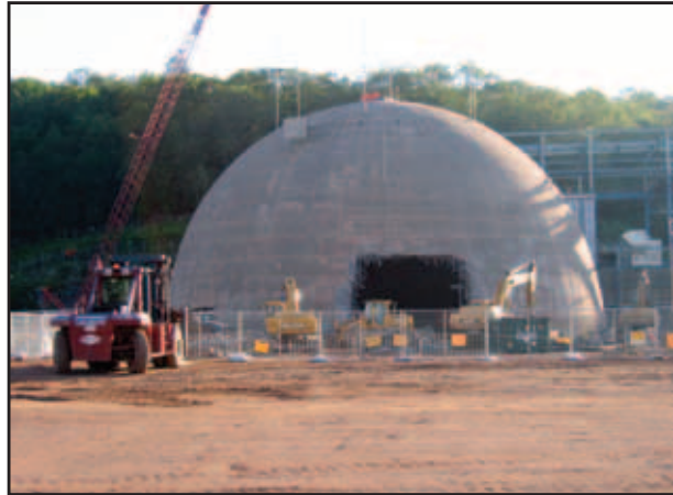
Demolition of the Connecticut Yankee containment building in summer 2006.
