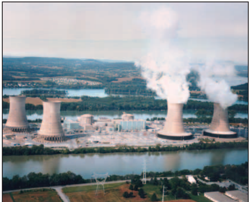
The Three Mile Island nuclear plant. Unit 2 is currently in postdefueling monitored storage status. Decommissioning of the damaged unit will take place concurrently with the decommissioning of Unit 1, sometime in the future.
