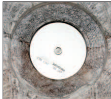
Horizontal boreholes in the walls of the WIPP disposal rooms will soon be used for the disposal of remote-handled transuranic waste. The article beginning on page 56 discusses how WIPP is preparing for that operation.
