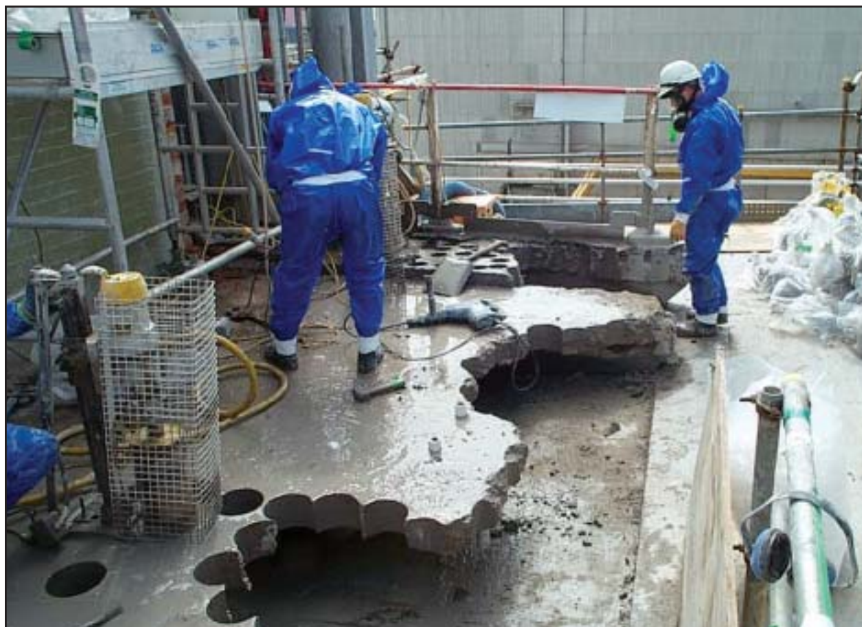
Wall demolition in progress.
