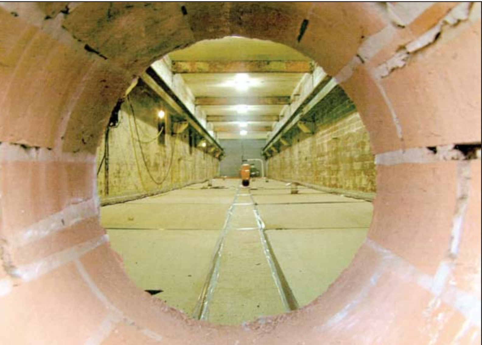
Looking into the waste-cleared tunnel through a vent connection hole.
