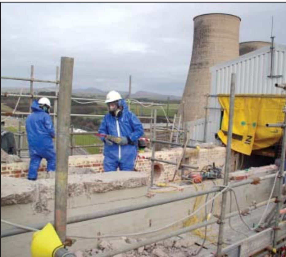
After workers completed cleanup of the tunnel annex, they began the next phase of work: demolition of the tunnel structure located on top of the 20.85-m facility. Demolition was completed using conventional tools of the trade.
