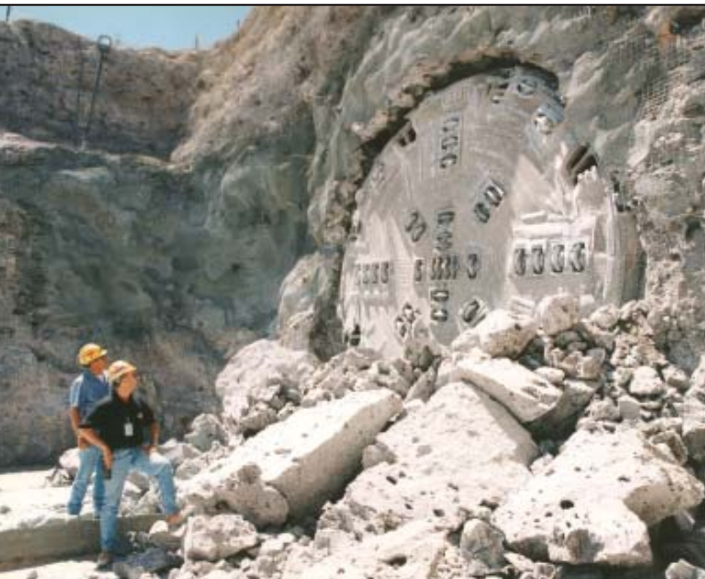
The tunnel-boring machine reached daylight in April 1997.
