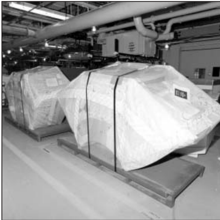
Disassembly lines of gloveboxes fill the aisles of Building 776/777, the converse of the assembly line created by Ford Motor Co.
