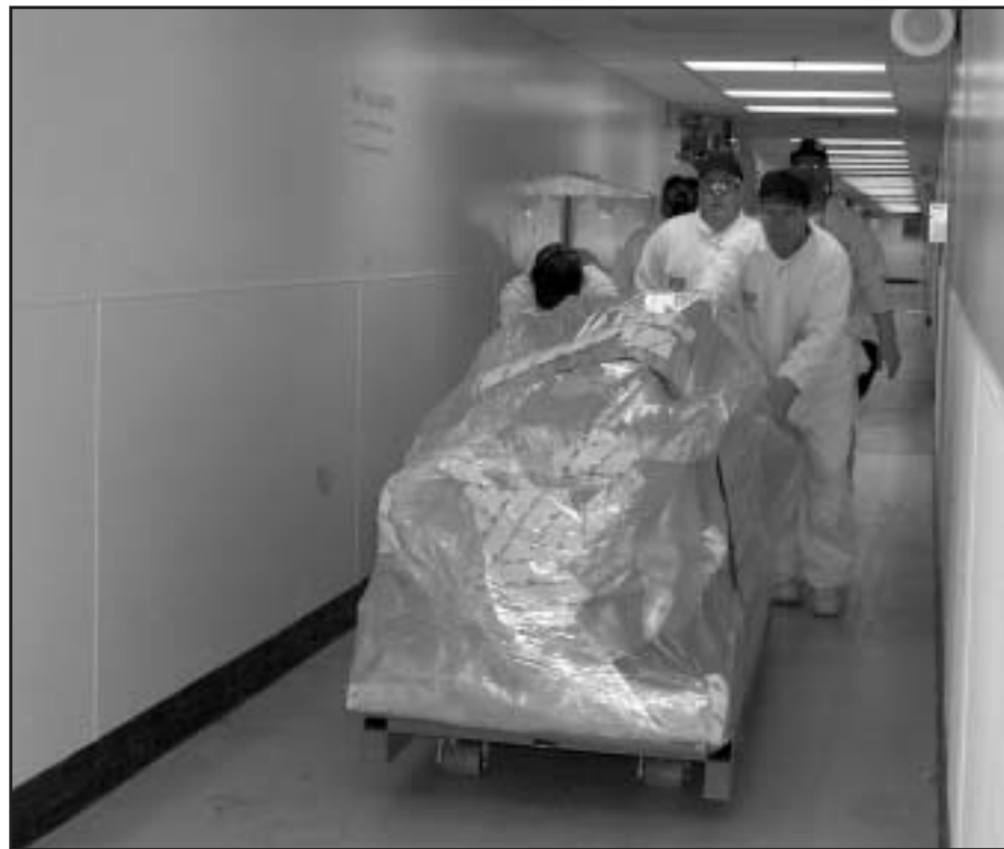
A Building 707 crew moves a decontaminated glovebox from the building.
