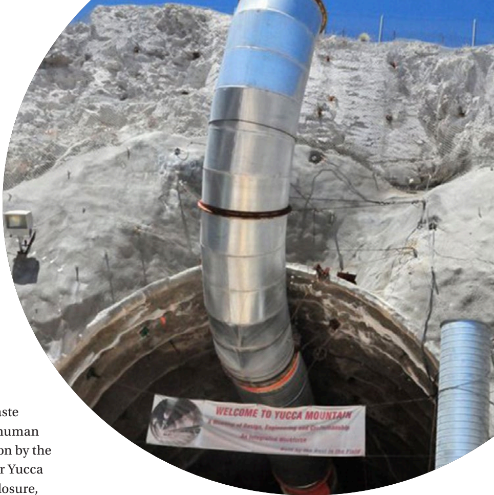
The Yucca Mountain mine portal.
