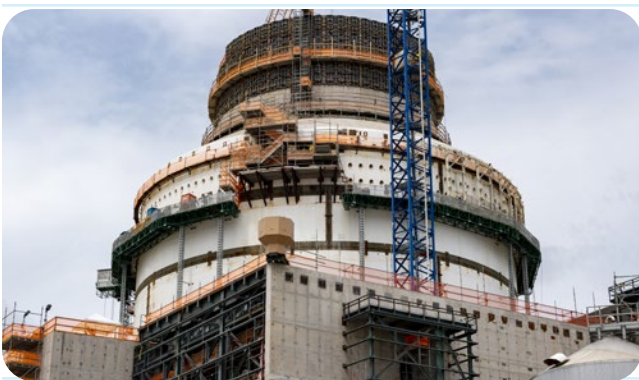
Vogtle-4 containment as it appeared in September. (Photo: Georgia Power)
