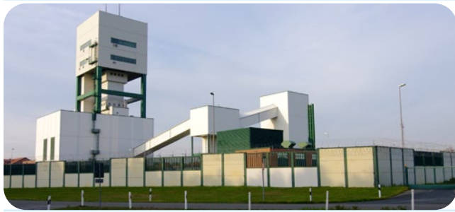
The headframe and buildings at the Gorleben salt dome in Germany. (Photo: Wikimedia Commons)
