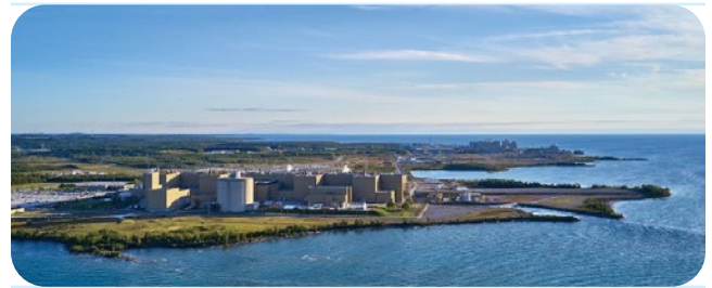
The Bruce nuclear power plant in Ontario, Canada. (Photo: Bruce Power)
