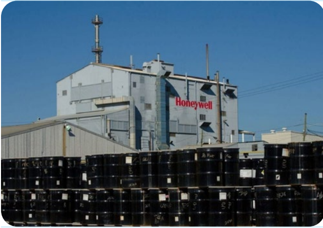
The Metropolis Works plant. (Photo: Honeywell)
