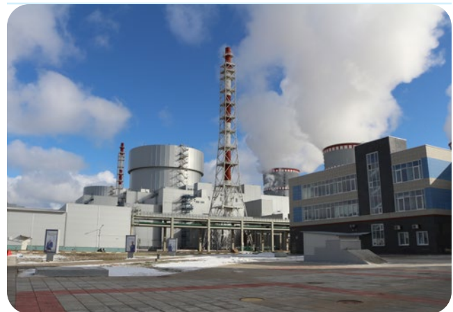
Unit II-2 at Russia's Leningrad plant. (Photo: Rosenergoatom)
