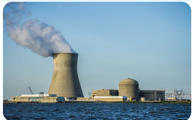
The Hope Creek nuclear power plant. (Photo: Peretzp)
