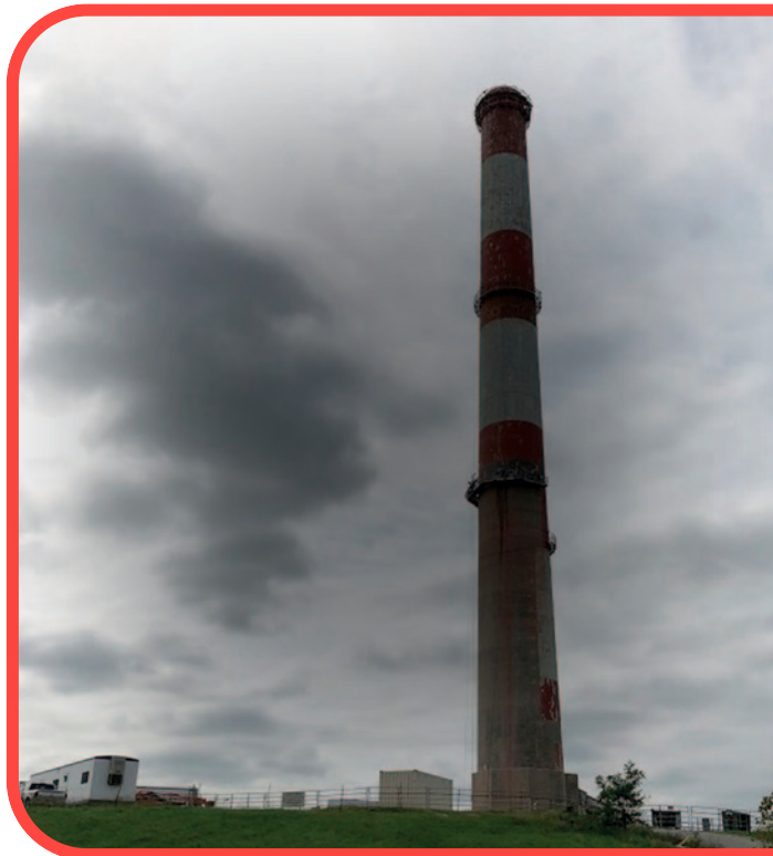
Below: The exhaust stack's distinctive red and white paint, which contained asbestos and lead, was removed late in 2020. (Photo: DOE)
