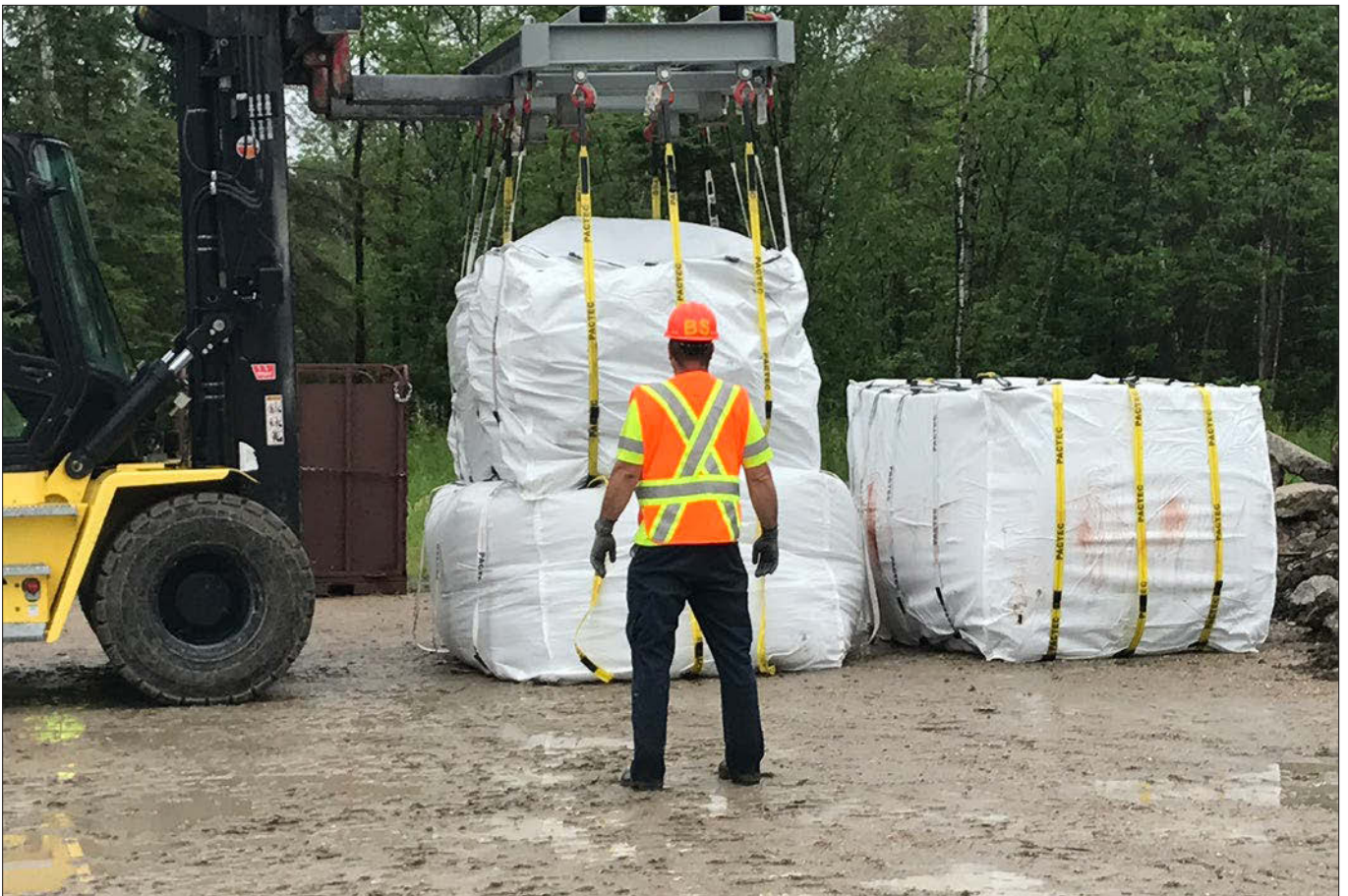
Pac-Tec LiftPacs are used to remove decommissioning debris from Canada's Whiteshell Laboratories.
