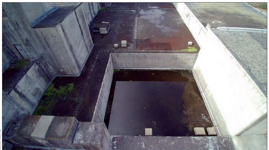
Potentially intrusive vegetative growth on an entombed nuclear reactor building.
