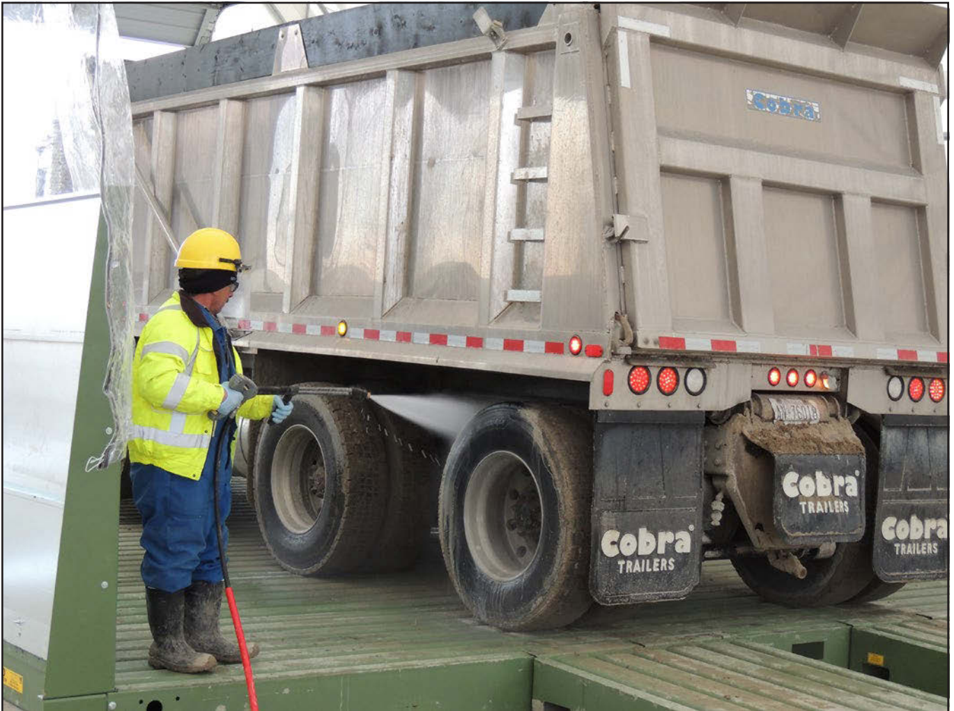
A truck is decontaminated at the Port Hope Project long-term waste management facility after depositing waste in the facility's baseliner storage cell.
