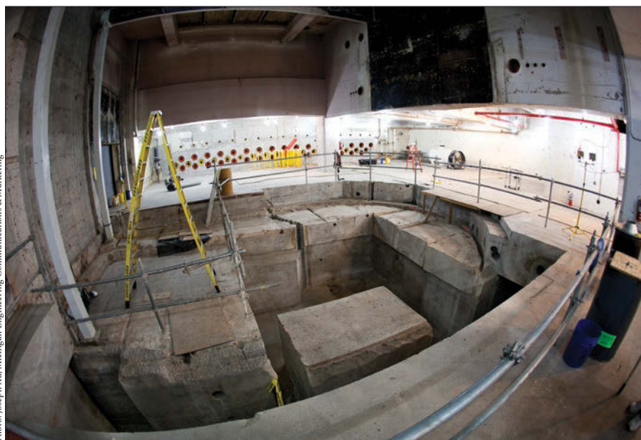
The old reactor space at the end of decommissioning.
