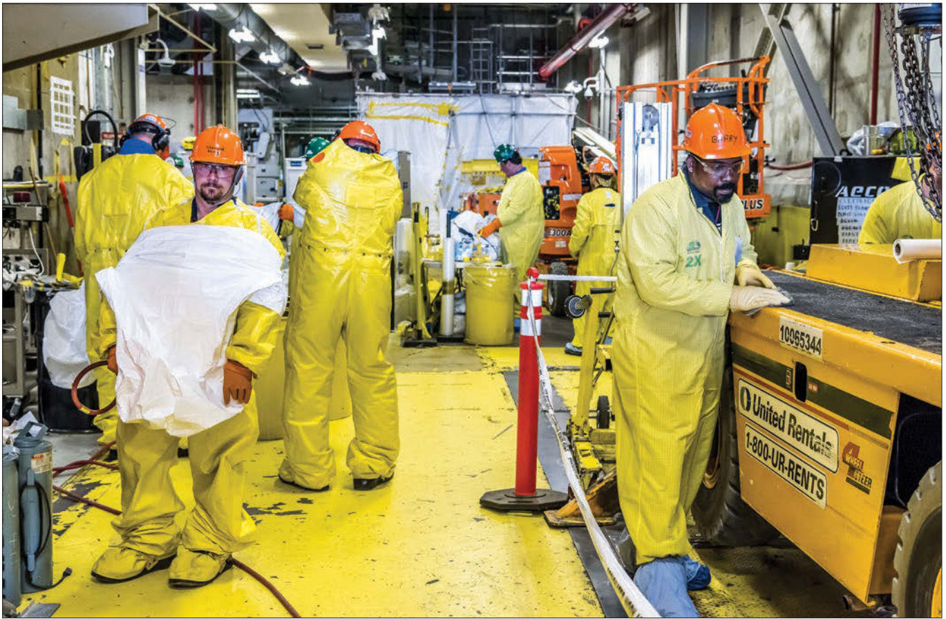
Yellow plastic suits are used to protect workers in potentially radioactive environments.
