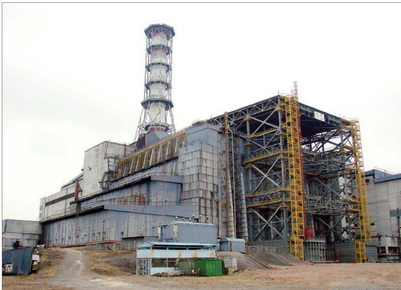
The photo above, taken on March 17, 2008, shows the stabilization work that was done at the deteriorating west wall of Unit 4's old shelter structure. Below is a view of that stabilized west wall taken on January 11, 2017, from inside the NSC structure.
