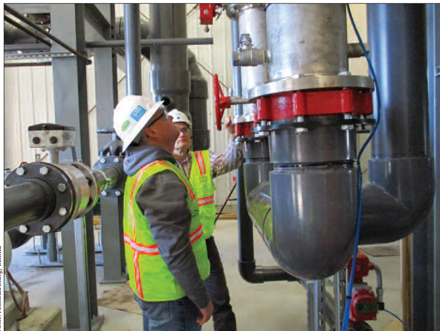
Crew members inspected ion exchange system valves and instrumentation at Strata Energy's Lance central processing plant in October.
