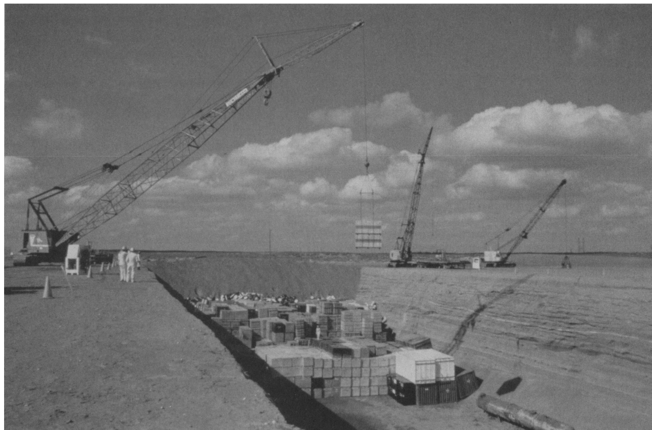
Fig. 22. Open-trench LLW site (Richland, Washington).
