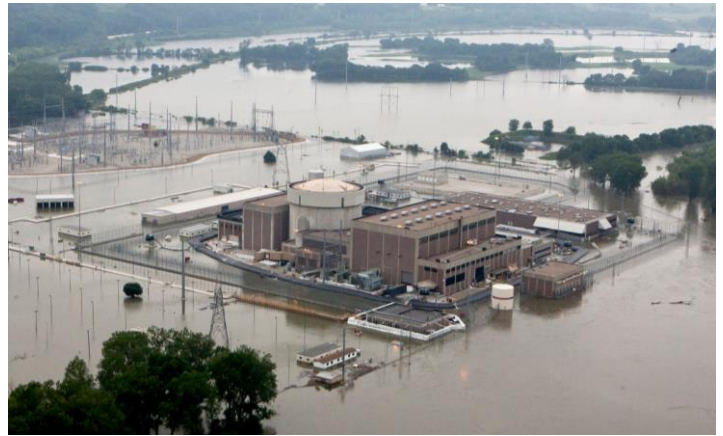
Missouri River floodwaters surround Nebraska's Fort Calhoun Station power reactor, June 2011 (photo: New York Times)
