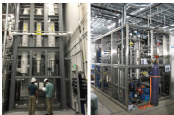
Figure 1: Exchange column (left); electrolyzer (right)
