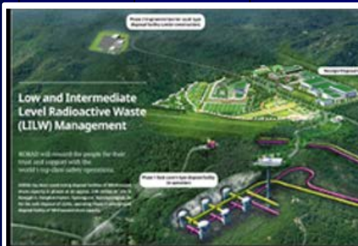
KORAD (Low- & Intermediate-Level Waste disposal)
