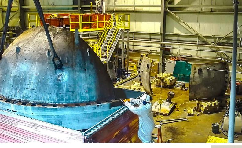
Vermont Yankee's segmented reactor vessel head is lowered into a custombuilt package for transportation and disposal. (Photo: Orano)
