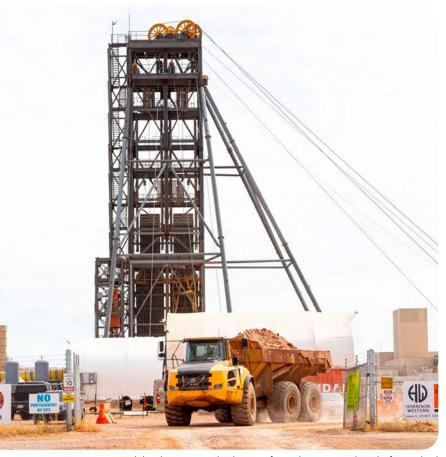
A truck hauls excavated salt away from the WIPP utility shaft, marked by a large aboveground steel headframe. (Photo: DOE)
