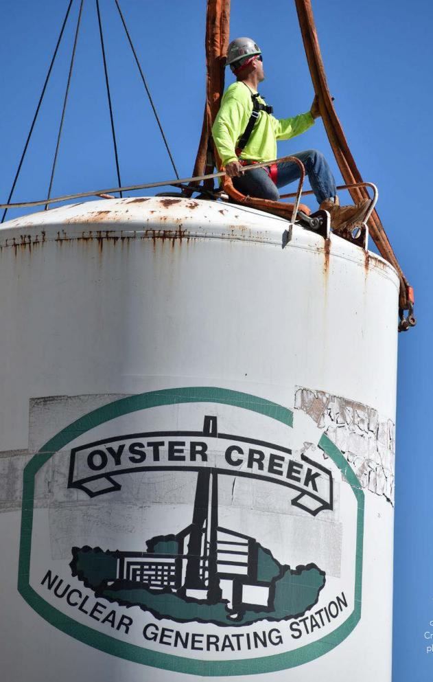
A rigger prepares a nitrogen storage tank to be taken down at the Oyster Creek nuclear power plant in New Jersey. (Photo: HDI)
