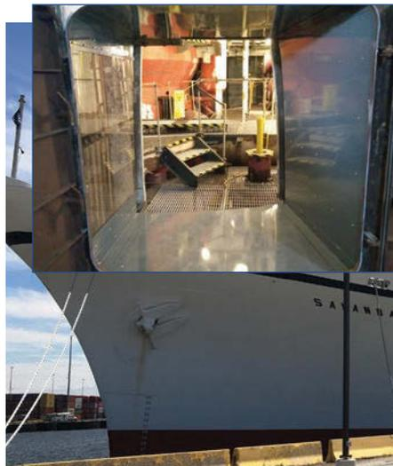
Inside the world's first nuclear cargo ship, we cut seven layers of steel plate, redwood and reinforced concrete to access the reactor compartment.
