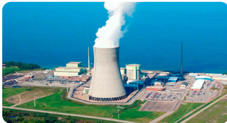
Nine Mile Point nuclear plant. (Photo: Constellation Energy)
